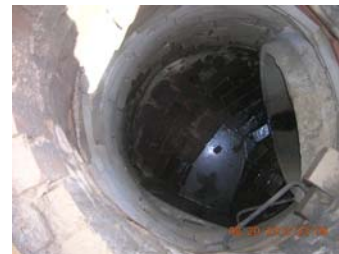
View inside Smith Street manhole
